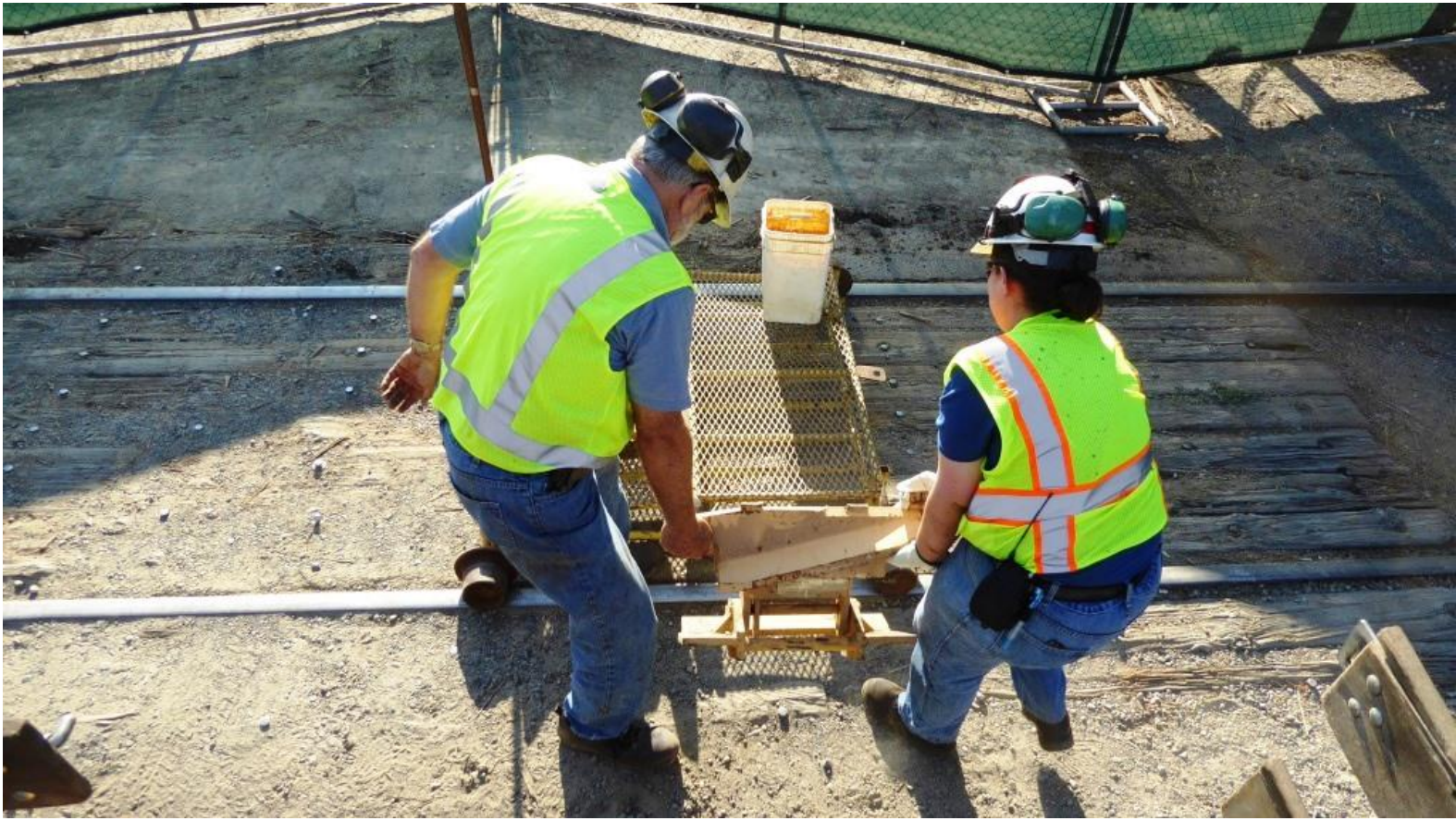
The derail, which weighs in excess of 100 pounds, is moved onto the track-cart
