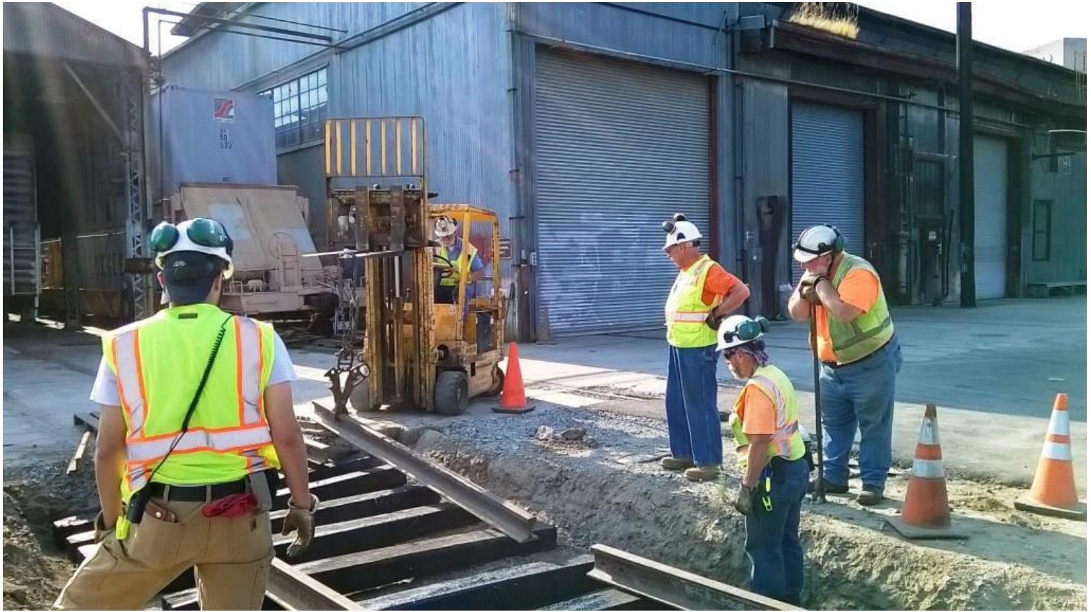
Alan on the forklift brings in that last stick of rail needed to connect the Firing Line to the Storage Track
