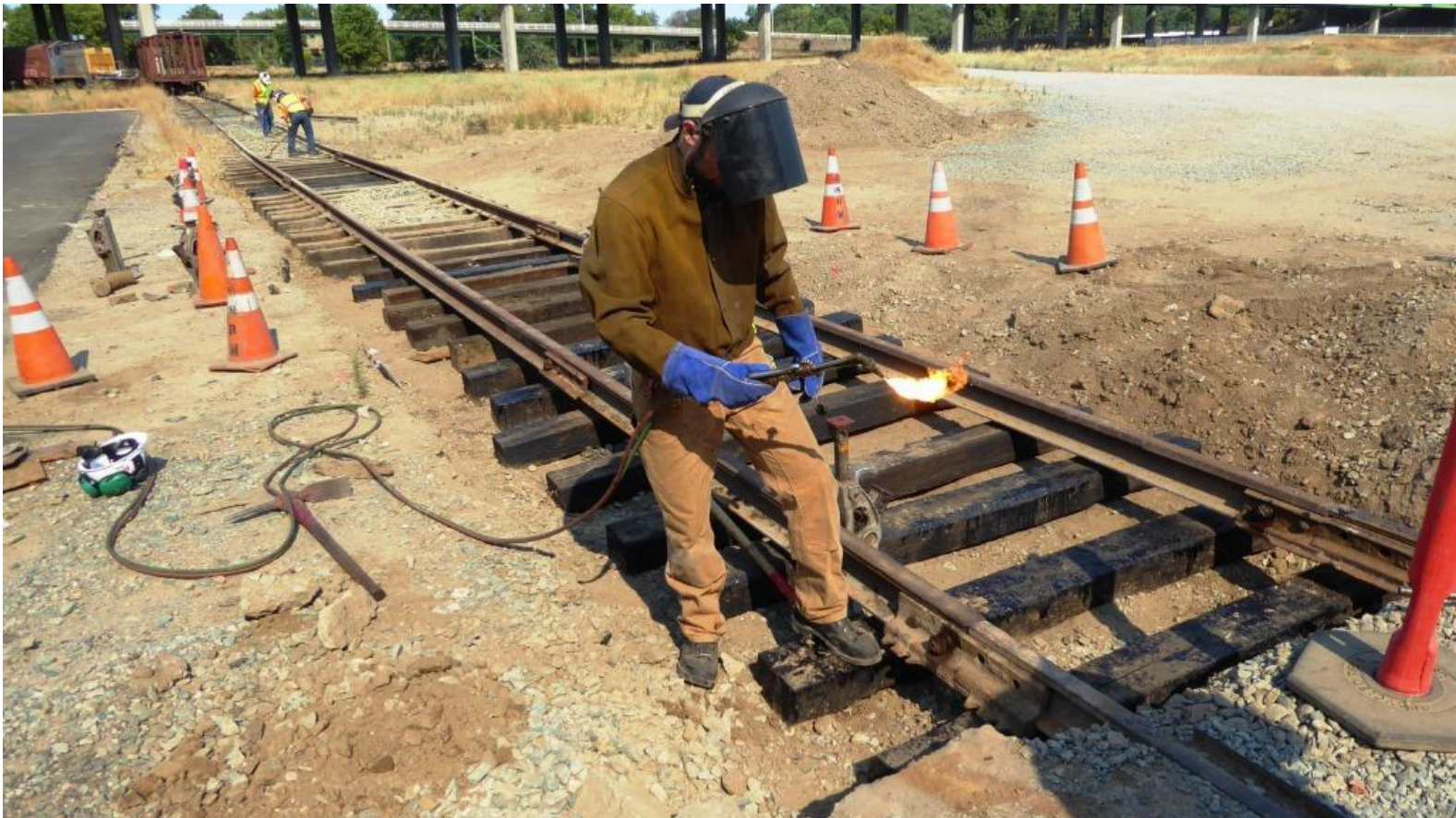
Kyle sparks-up his acetylene-torch to blast bolt-holes through the rails
