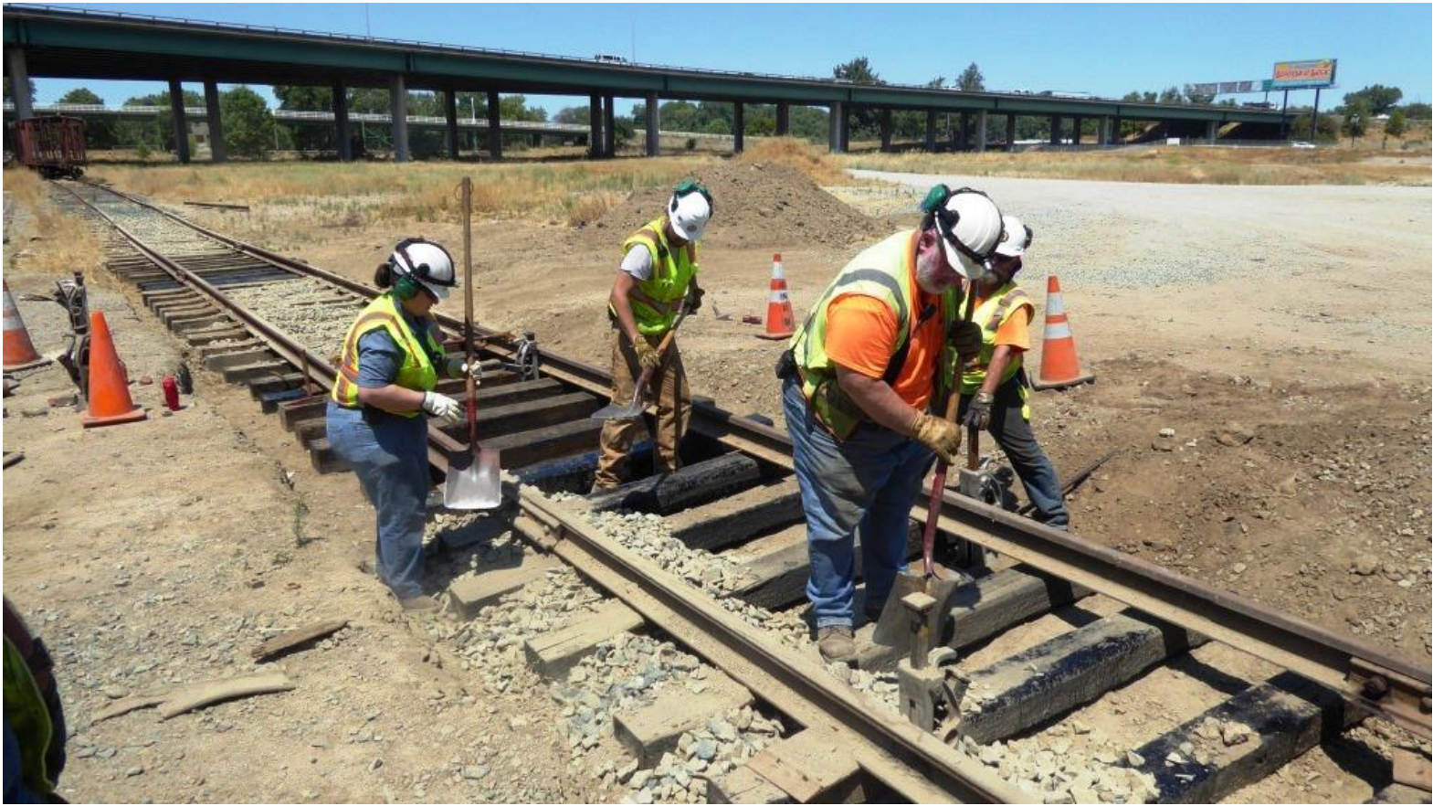
Heather, Kyle, Frank, and Joe spread the rock about the rails
