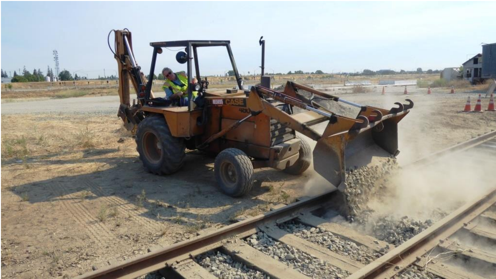
Chris rotates the backhoe's bucket to pour the ballast-rock onto the track
