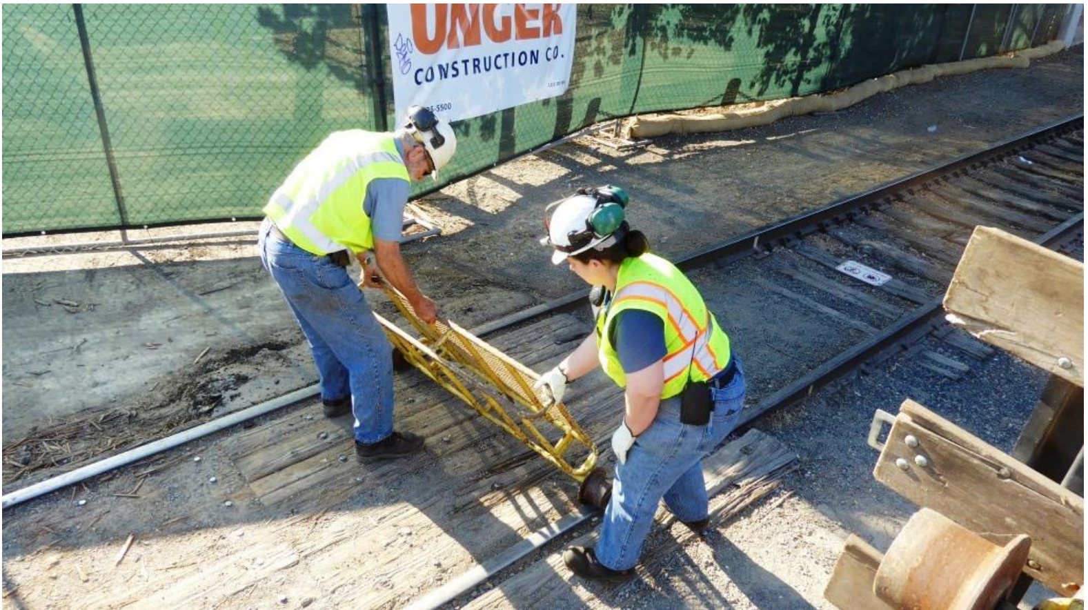
Alan and Heather set up a Nolan track-cart for transporting a derail
