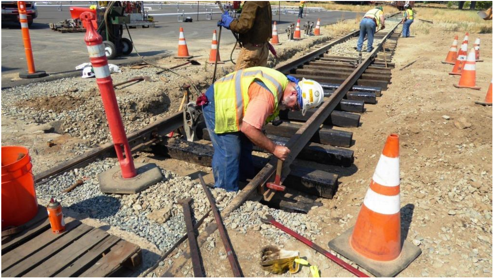
Mike breaks-out any slag that may remain from the newly torch-cut bolt-hole
