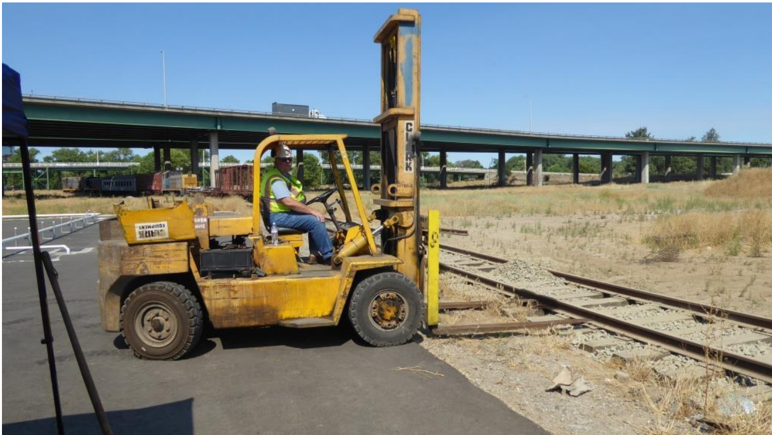
Chris uses the 15,000-lb forklift to line the track
