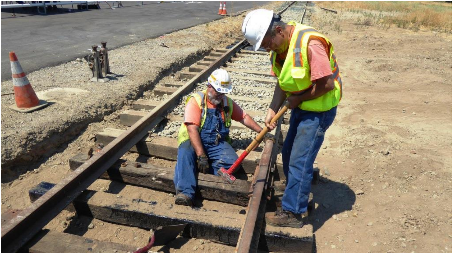
The shoulder of the bolt was slightly too big for the hole so, Mike says, "Whack-it with a capital 'W'!" as John whacks the bolt through
