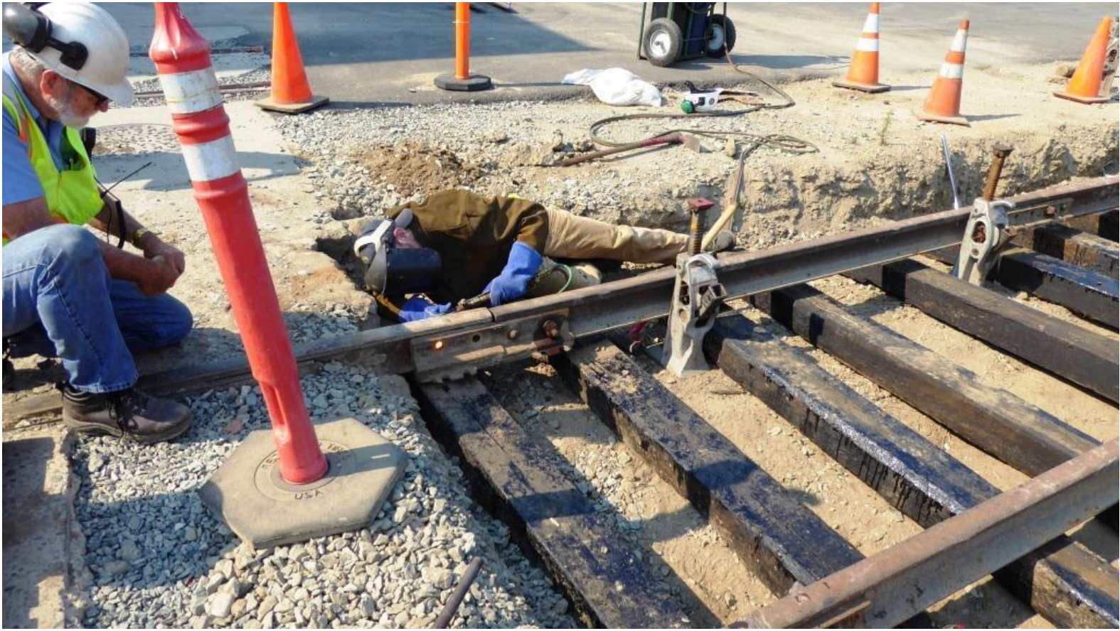
Alan observes as the heat from Kyle's torch glows through the rail
