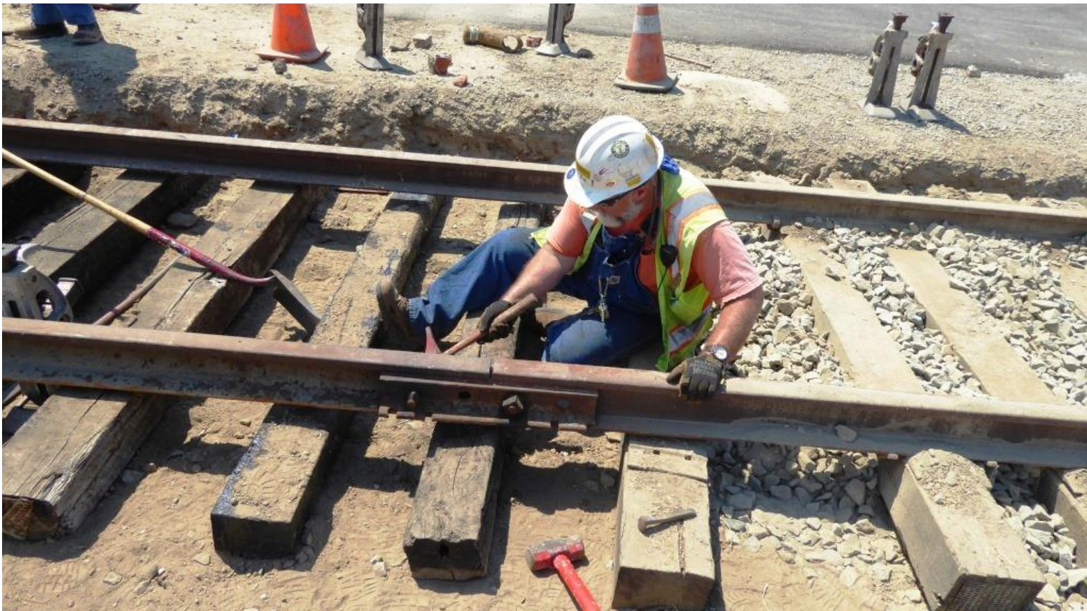
Mike knocks a bolt through the newly cut hole
