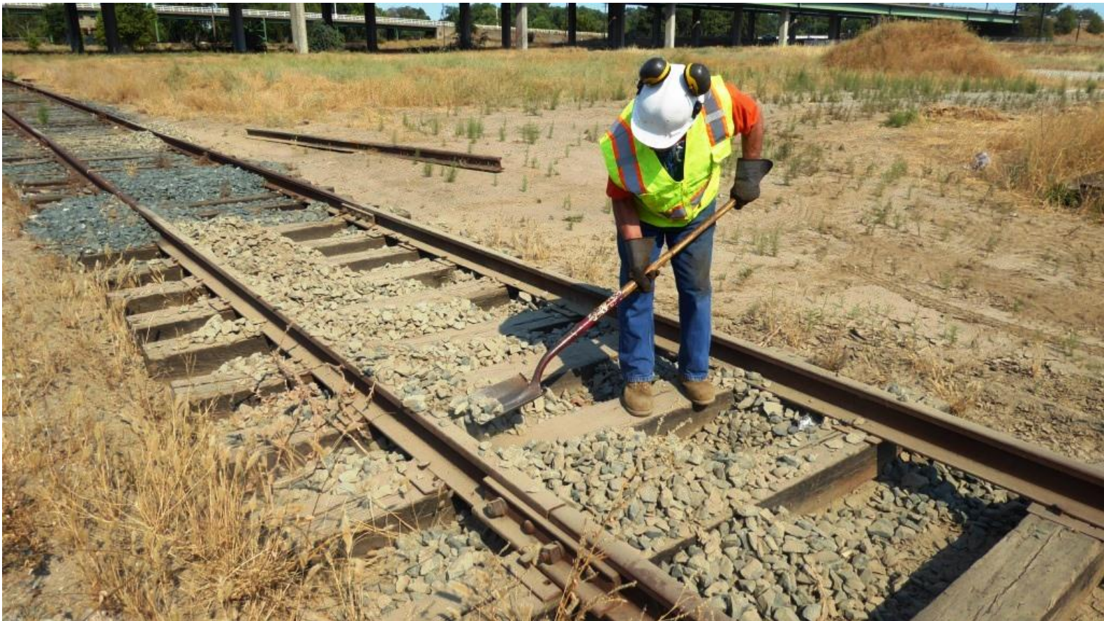
Clem, the human ballast regulator, spread ballast-rock about the track
