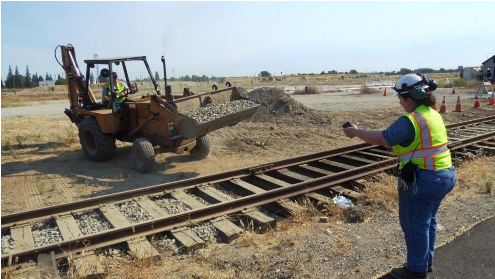
Heather guides Chris on the backhoe as to where to drop the rock
