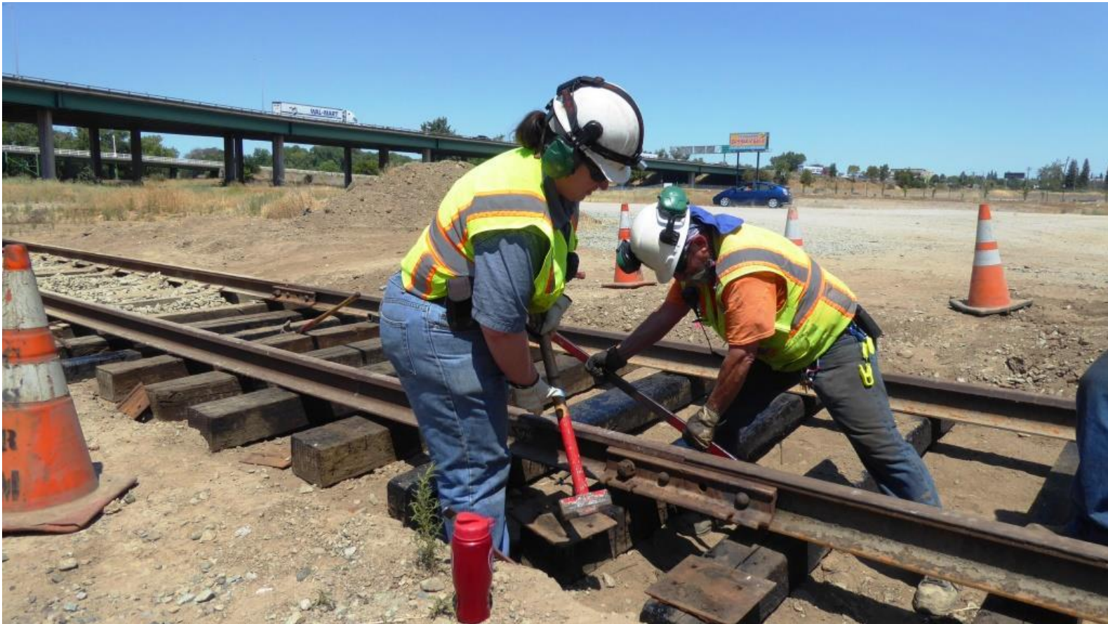
Heather hits the bolt-head with the sledge as Joe tightens it down
