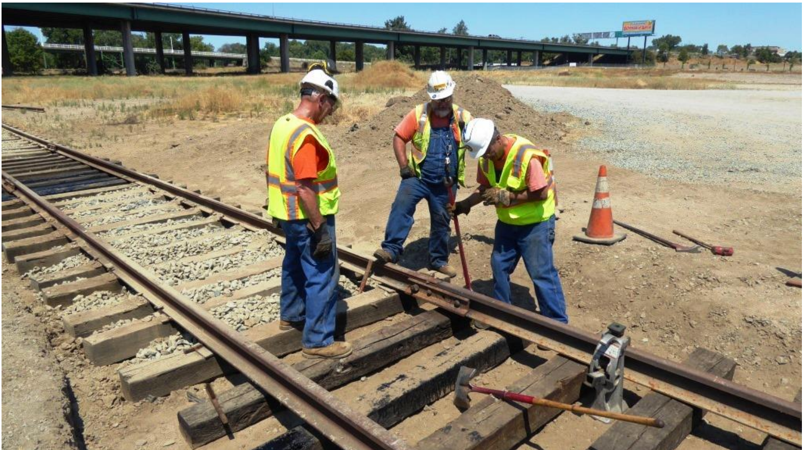
Now John tightens the nut on the whacked bolt
