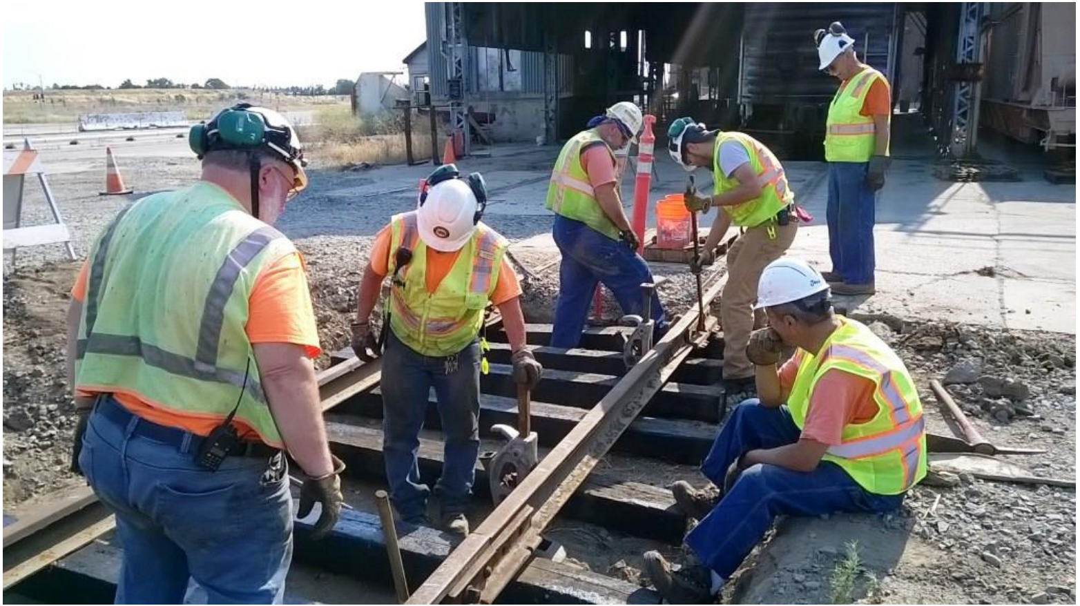
Using a track-jack, Joe raises the west rail even with the east as Kyle pulls on the track-wrench tightening bolts
